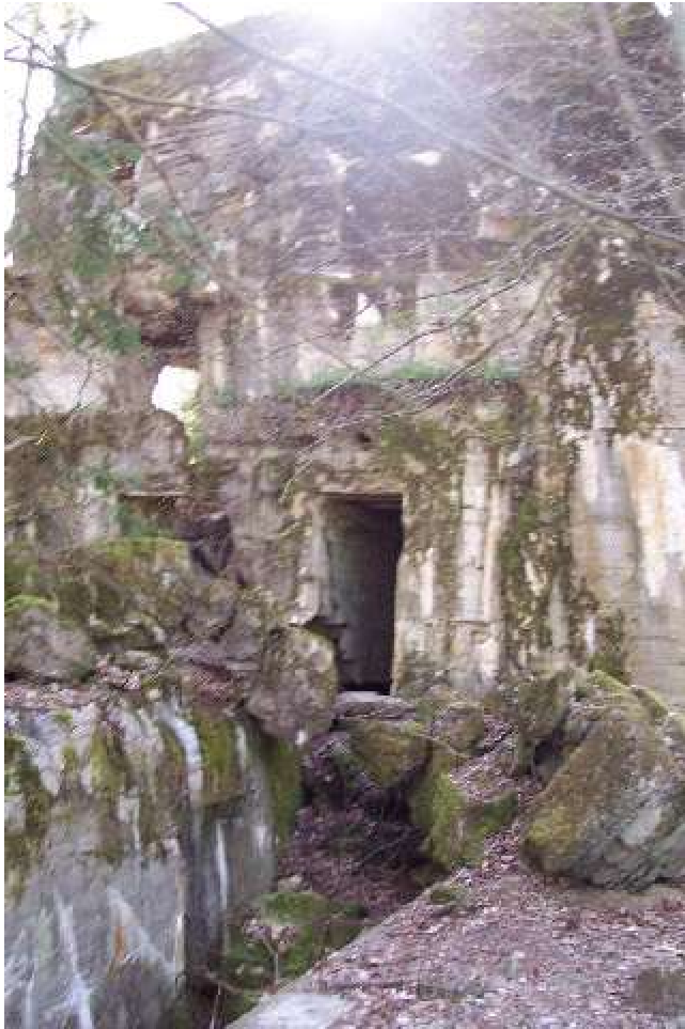
Fig. 62: Concrete Bunker at the “Wolf’s Tail”
